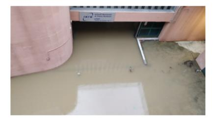
All Tier-1 doors are watertight Height of water outside: 50 cm Height of water inside: 10 cm (on floating floor) for a total volume of ~500 m<sup>3</sup>
